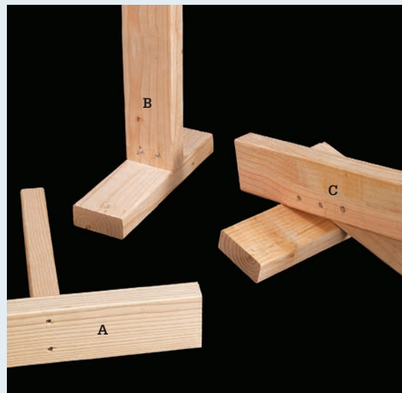
Endnailing (A), toenailing (B), facenailing (C).
