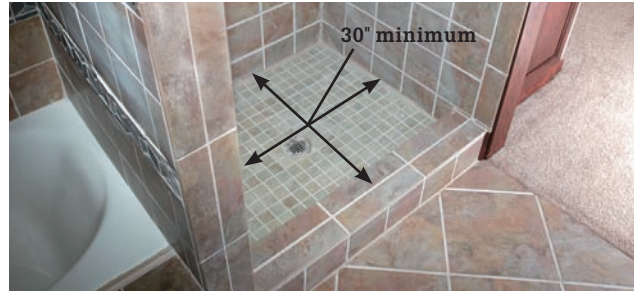
A sufficiently large shower stall is more than a convenience—it is a safety issue.
