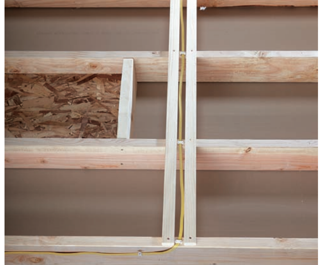
Use wood or other substantial guards to protect NM and UF cable installed on top of ceiling joists within the protection area.
