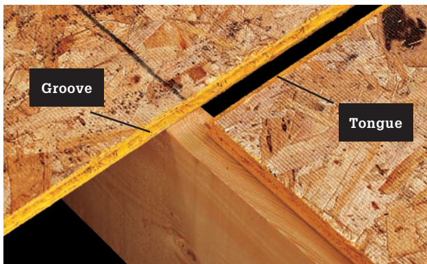
Support edges of floor sheathing with tongue-and-groove edges.
