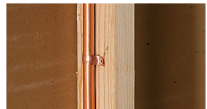
Provide vertical support for pipes running parallel to wall studs. Install supports according to Table 32.
