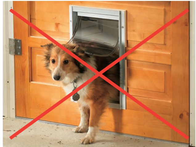
VIOLATION! DO NOT install pet doors in doors that separate the garage from the dwelling.
