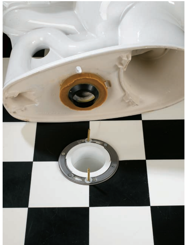
The closet flange and O-ring seal the plumbing connection. The closet flange does not support the toilet.
