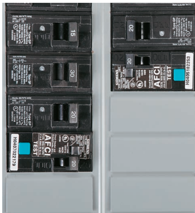
A combination ARC-fault circuit breaker detects sparking (arcing) faults along damaged energized wires and detects these faults between wires. A branch ARC-fault circuit breaker only detects arcing faults between wires.
