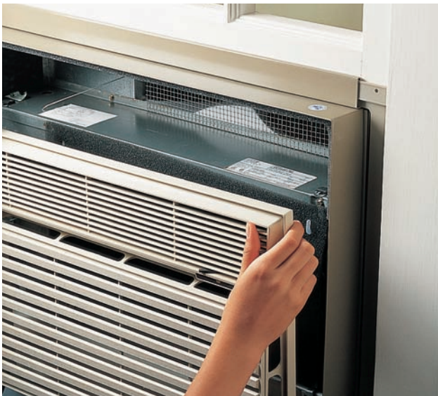
Air-conditioner load ratings can be found on the nameplate.
