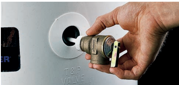
T&P valves should be installed on your water heater prior to placing the appliance in position. Many water heaters today come with the T&P valve preinstalled.
