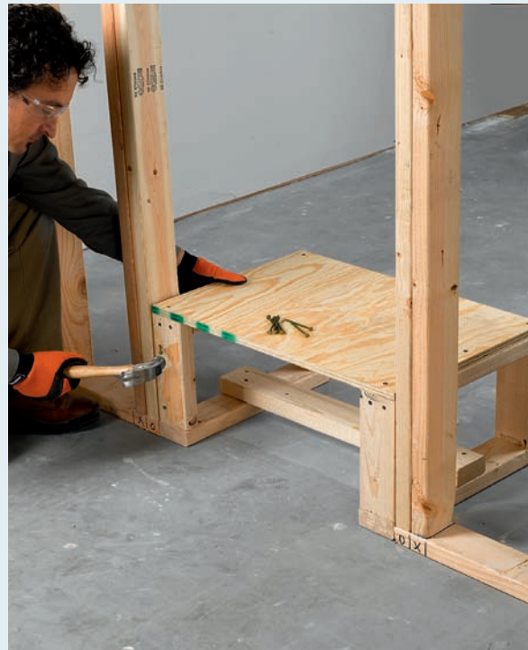
Factory-built fireplaces (including direct-vent and vent-free gas fireplaces) typically require structural support. If the fireplace is recessed into a wall, structural support is in the form of a mounting platform located on the other side.
