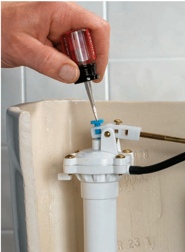
The water inlet of a fill valve should usually be above the tank's water line to reduce backflow of wastewater into the drinking water system.
