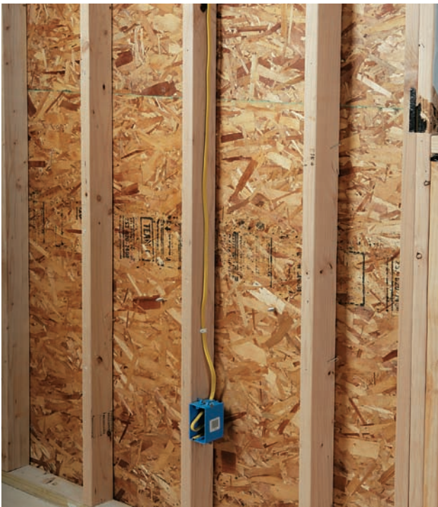
Support NM and UF cable at least every 4½ ft. Cable on top of ceiling joists is considered supported.
