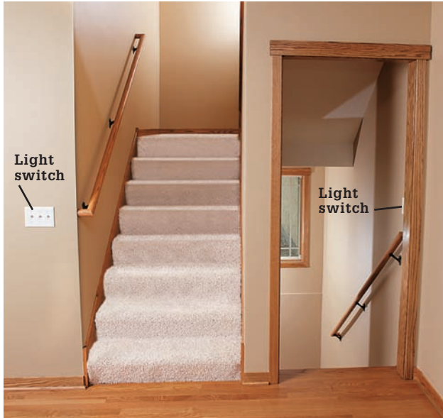
Install a light switch at the top and bottom of stairways with at least six risers.
