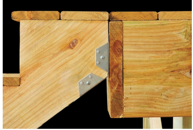
Attach stringers to support using a hanger, not just nails.
