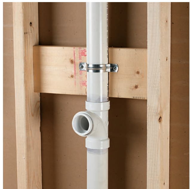
Individual vents are the easiest to install. They protect one fixture.
