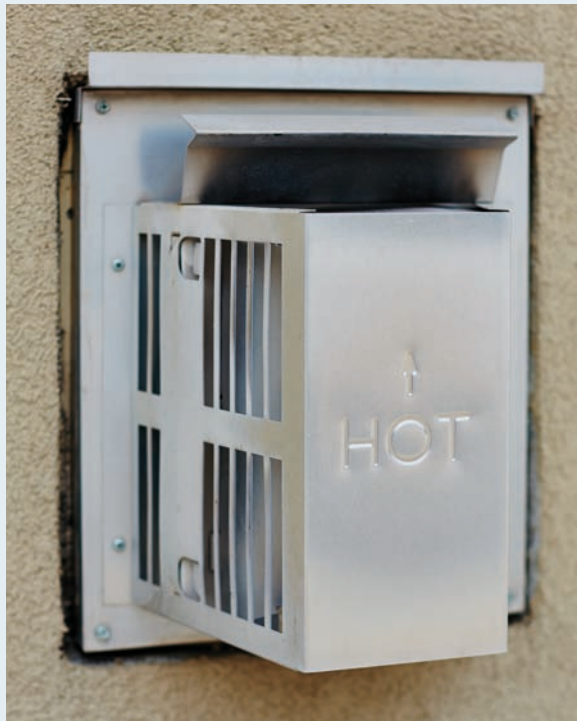
Vents for gas fireplaces must have a protective termination cap (supplied by manufacturer).
