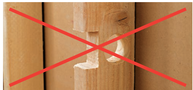
VIOLATION! Do not locate a notch and a hole in the same part of the stud.
