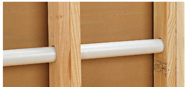
Double two load-bearing studs if the holes are not more than 60 percent of their actual depth.
